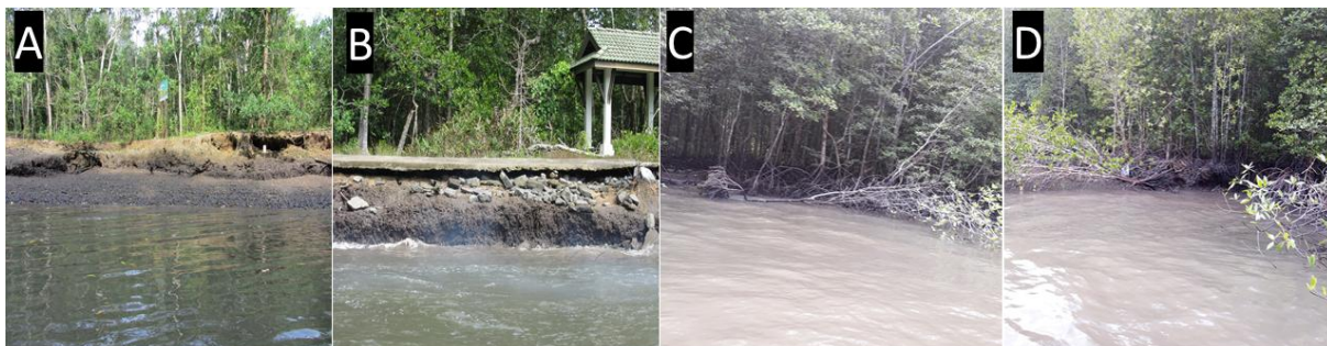
Figure 1. Riverbank erosion (A,B) and mangrove collapsed (C,D) at Kilim River.
