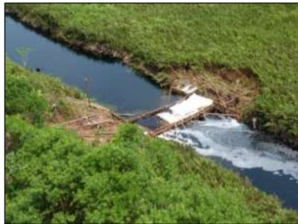
Figure 2. Canal blocking installed at RMFR
