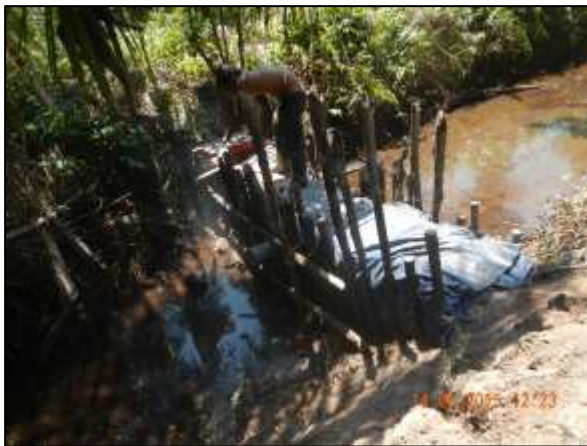
Figure 1. Canal blocking installed at RMFR
