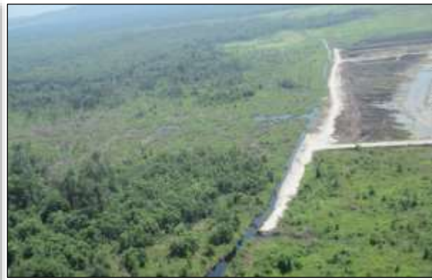
Figure 4. Clay dyke constructed between the degraded peat swamp forest and clay mine area
