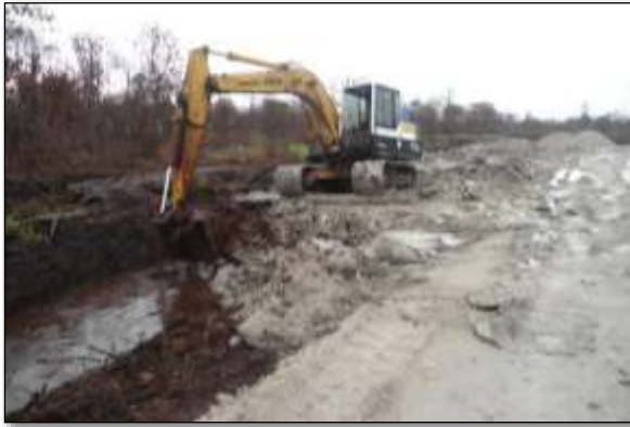
Figure 3. Clay dyke constructed between the degraded peat swamp forest and clay mine area
